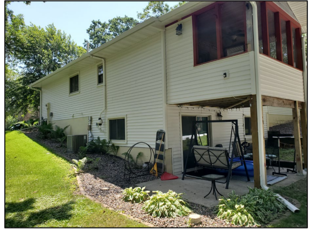
Home after using Homeowner Rehabilitation Program
