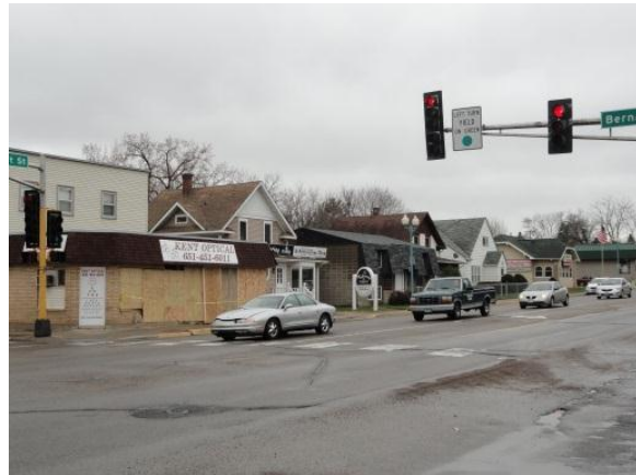
Commercial building at SE corner of Robert and Bernard Streets
