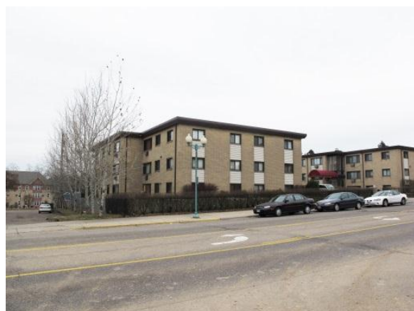
Twin Pines Condominiums (east side of Robert Street between Haskell and Bernard Streets)
