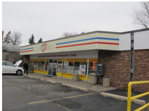
Convenience store at NW corner of South Robert and Annapolis Streets
