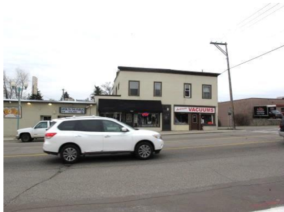
Looking east from South Robert Street at the existing commercial building
