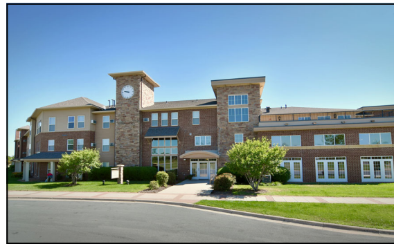
Vermillion River Crossing, Farmington
