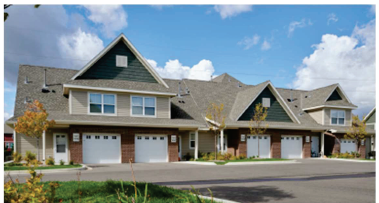
BLDG. TYPE 1,3 AT PRESTWICK PLACE IN ROSEMOUNT, MN
