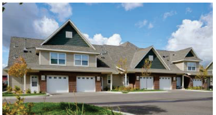
BLDG. TYPE 1,9 AT PRESTWICK PLACE IN ROSEMOUNT, MN
