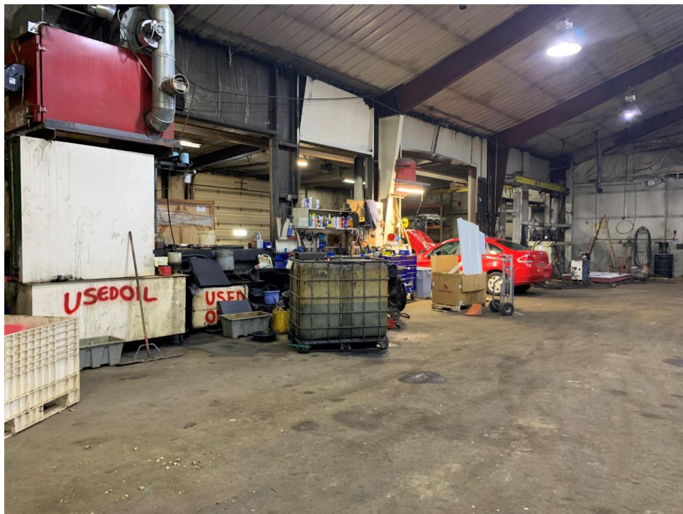
Used oil furnace and used oil tote storage.
