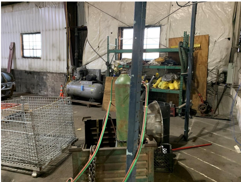
Welding storage area in newer garage
