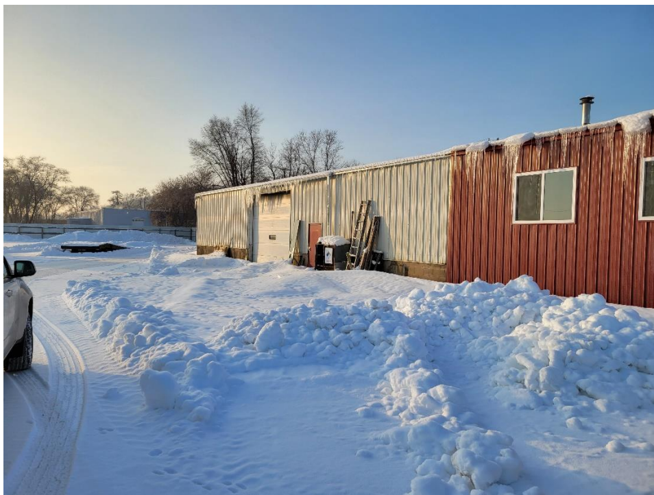
Subject Property building facing southwest.
