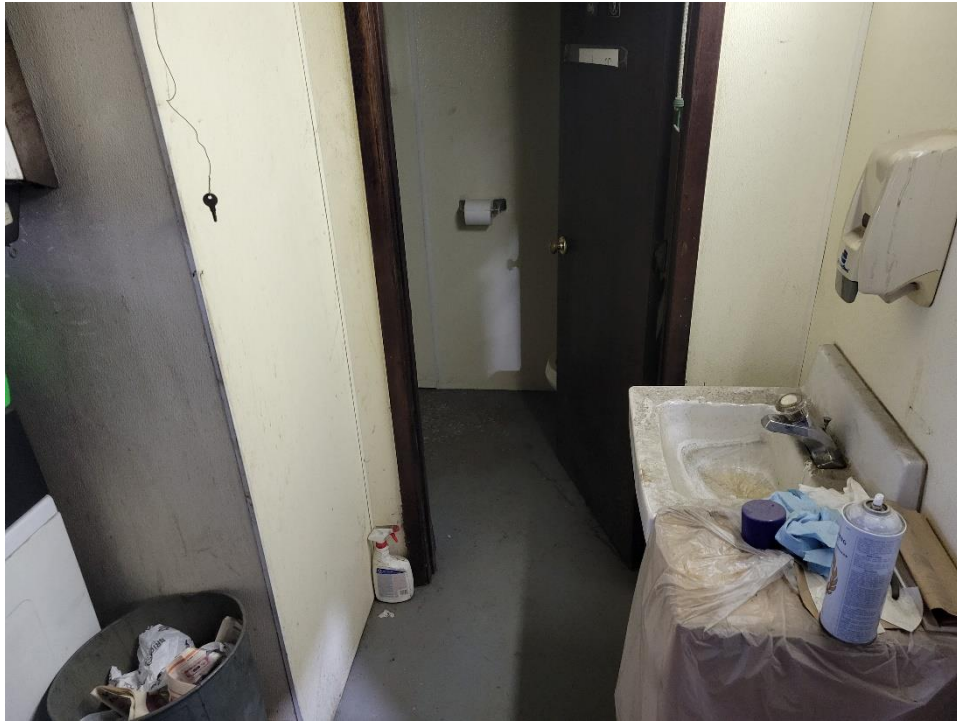
Bathroom in Subject Property building.
