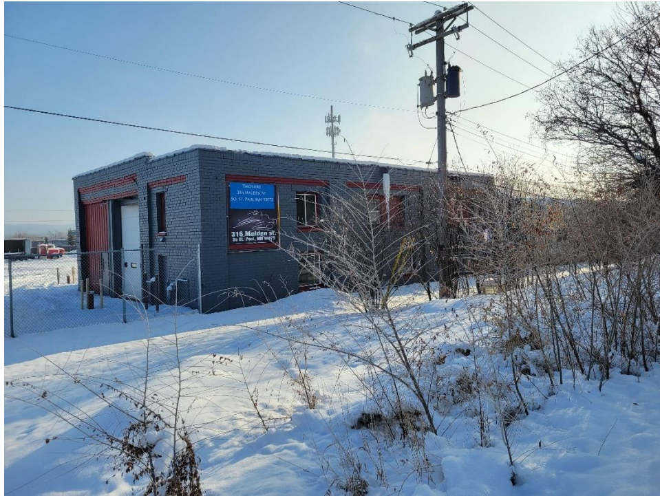
Subject Property building and pole-mounted transformer, facing southeast.
