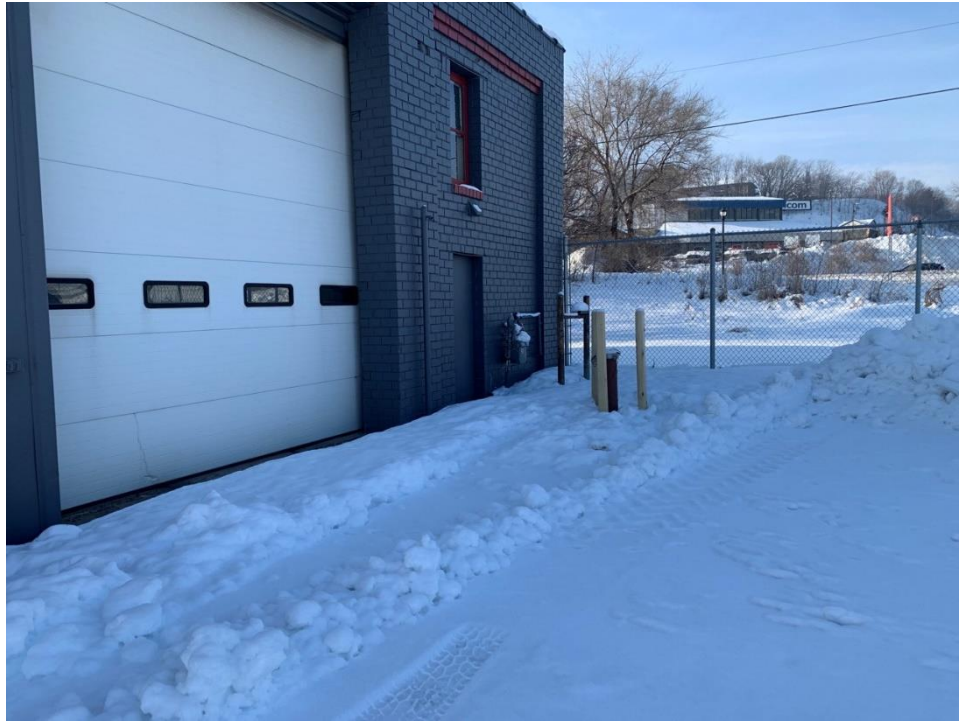
Old garage entrance. 1 of 4 monitoring wells on Subject Property.
