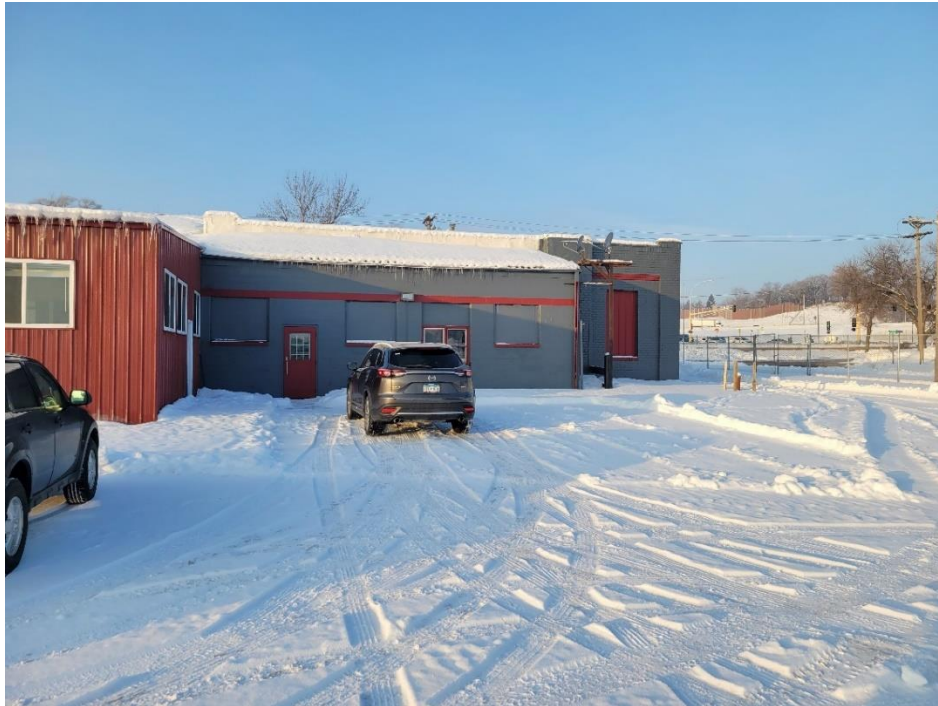
Subject Property building. Facing west.
