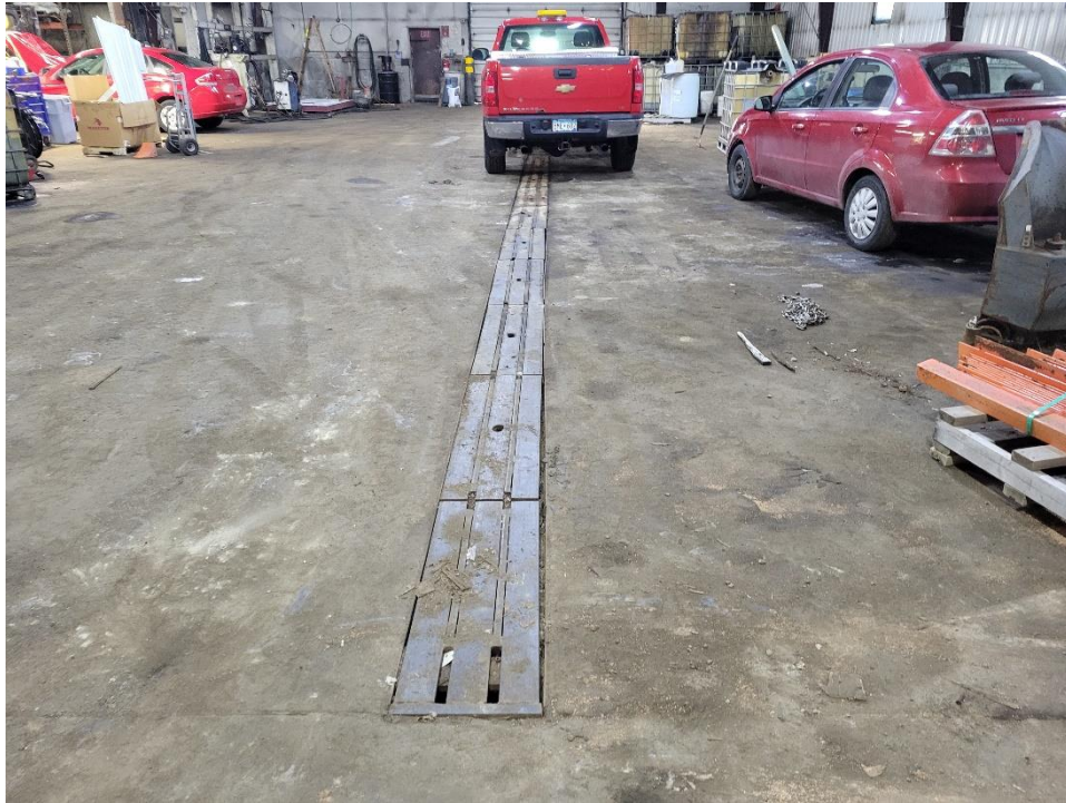
French drain connected to oil water separator in new garage
